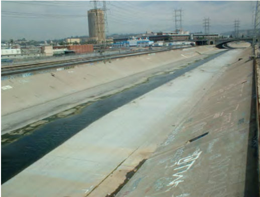
写真-6 1st Street 橋上流方向
